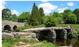
The Old Clapper Bridge, Postbridge
